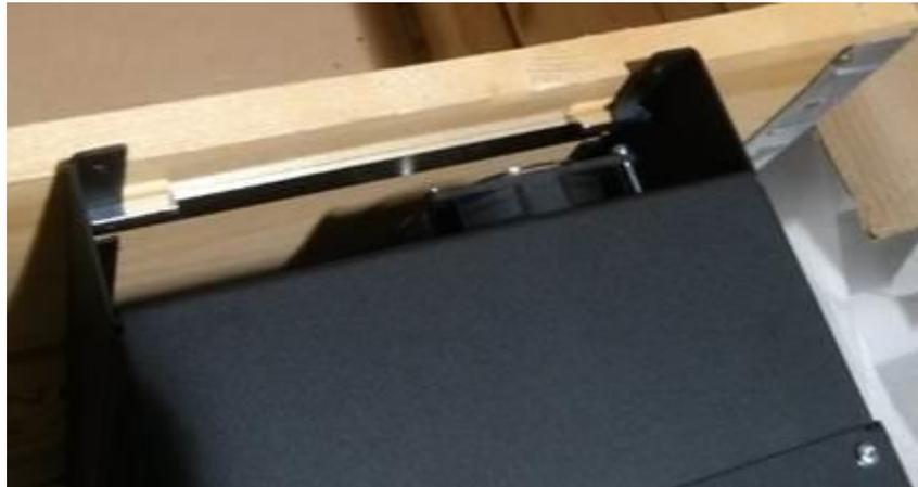
Once the charger is hanging from the bracket, mark the position of the lower charger mounting holes on the wall.
